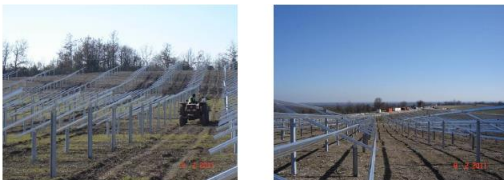
Figure 18: Montage des structures porteuses
